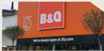
c.30% space reduction achieved at B&Q Canterbury – March 2021
