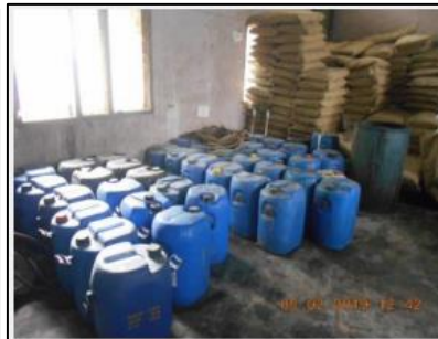
Non-compliance: No secondary containment for chemicals
