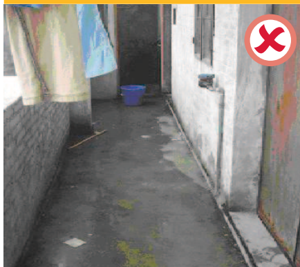
Poor accommodation facilities
